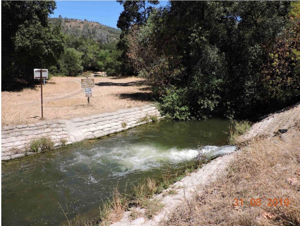
Photo 9. Release from the downstream pipeline below Anderson Dam on 31 August 2019. Releases to Coyote Creek for most of the summer were from mid-level Anderson Reservoir water released immediately below the dam and through the downstream hydro pipeline below the dam.
