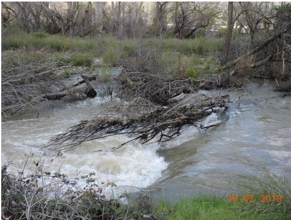
Photo 4. The stream gage weir at Coyote Ranch Road on 10 February 2019 at a flow of 350-400 cfs through several channels. The site was passable from February through mid-March, but not at 32 cfs on 1 April 2019. It is a major passage impediment at lower flows because of boulders at the base of the weir that interfere with jumping.
