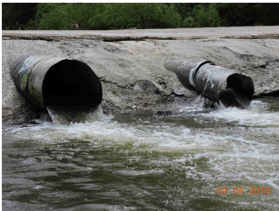
Photo 8. Singleton Road Crossing after stream flows had dropped further to about 40 cfs on 1 April 2019. Adult steelhead passage would have been possible through the culvert on the left.
