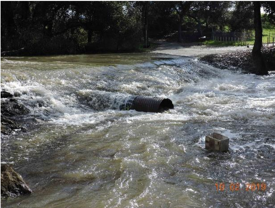
Photo 6. Singleton Road crossing of Coyote Creek on 10 February 2019, during February through mid-March stream flow of about 500-600 cfs. High velocity in the culverts would have blocked passage, but the depth of flow (and moderate velocity) over the apron may have allowed adult steelhead upstream passage over the apron and submerged crossing.
